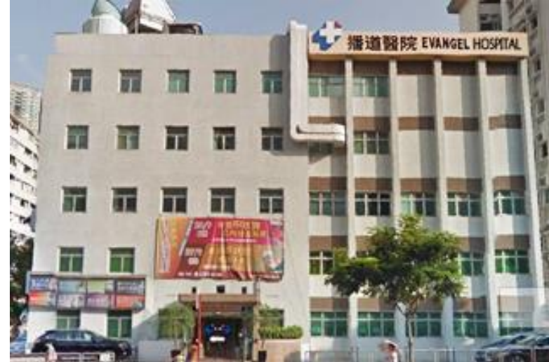
Before installation of elevator
