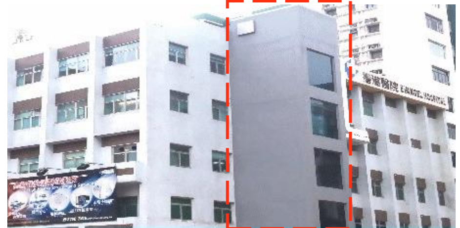
After installation of elevator
